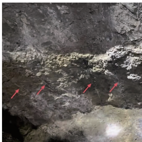
(a) Air-uncoupled charge blasting
