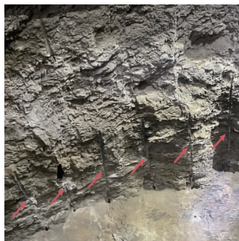
(b) Water-uncoupled charge blasting
