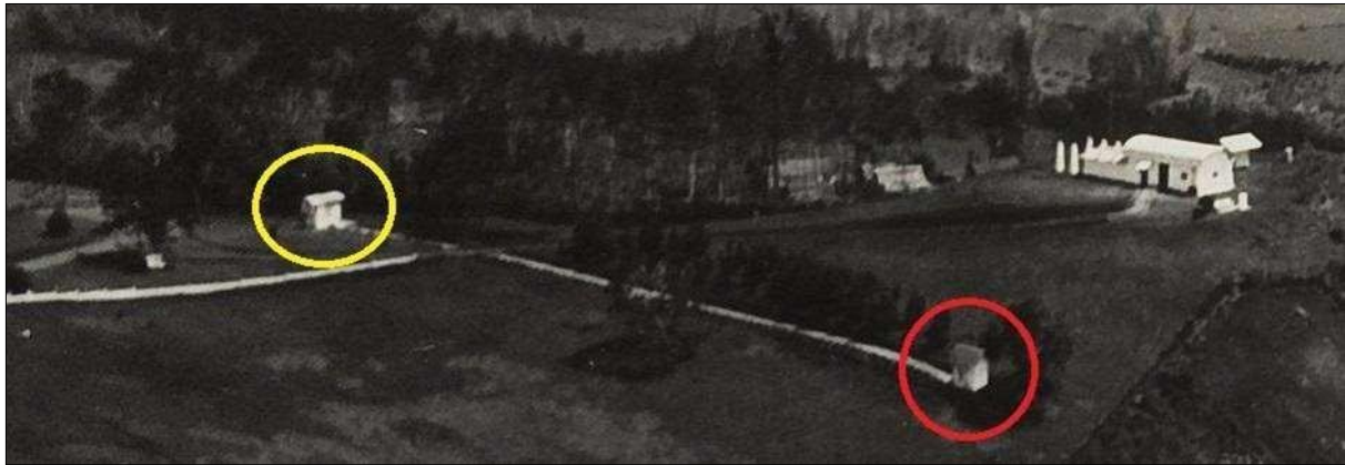
Figure 7: The transit telescope building with the white meridian track to the south, circa 1928. The yellow circle marks the transit telescope building, while the red circle marks the meridian pillar to the south, as a collimator. Above and to the right is the building for the Bamberg Astrophotographic Refractor with its sliding roof (courtesy: Leiden University Libraries, Luchtvaart Afdeeling Koninklijk Nederlandsch-Indische Leger, KITLV 38859, http://hdl.handle.net/1887.1/item:910823 ).
