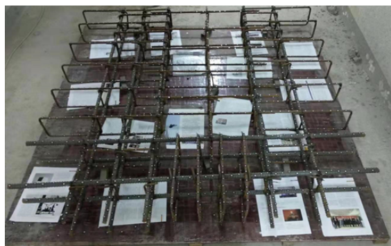
图 4 粘贴标记点后的钢筋骨架 Fig. 4 Reinforcement skeleton after pasting the marked points
