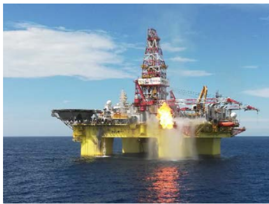
图8 海洋石油982钻井平台 Fig.8 Haiyang Shiyou 982 Drilling Platform
