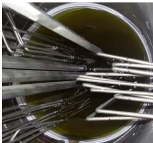
图 13 冷冻壁局部破损 Fig.13 Local damage of frozen wall.
