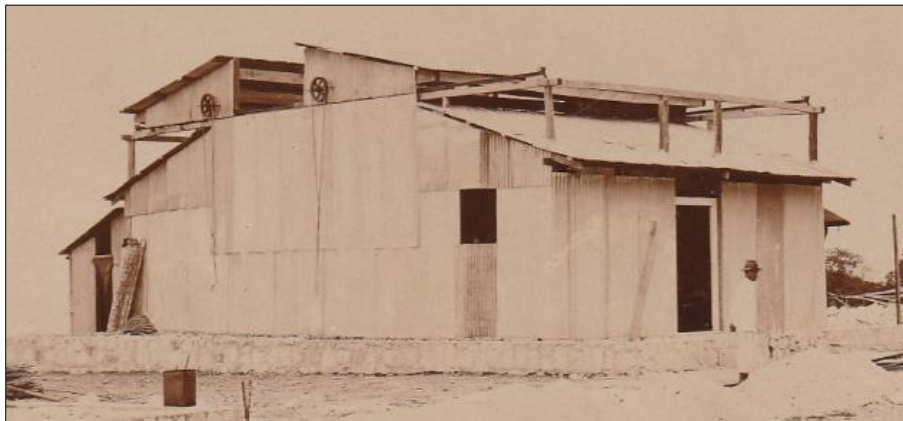
Figure 9 (right): Erecting the observatory building (courtesy: John Hunt).
