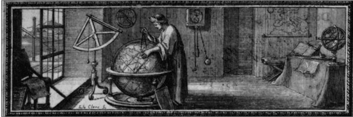
Figure 1: Drawing from Richer's Observations Astronomiques et Physiques Faites en l'isle de Caïenne (Paris, 1679). Most of the astronomical instruments used by Richer are shown, including one of Isaac Thuret's (1630–1706) pendulum clocks (artist: Sebastian Le Clerc; Creative Commons Attribution-ShareAlike License).
