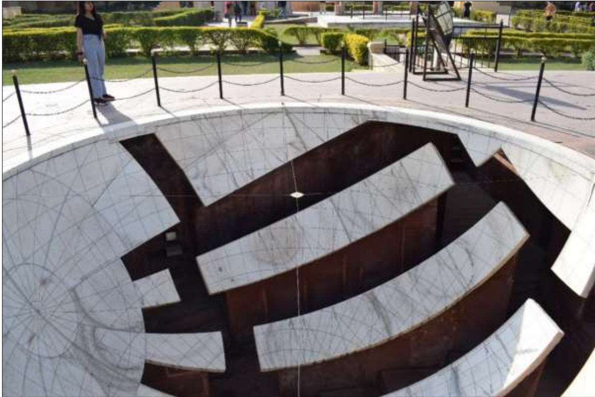
Figure 6: The Jayaprakash yantra ; two strings are tied along the E–W and N–S directions holding the ring on the top. The shadow of the central ring gives the location of the Sun, since the bowl is graduated as a mirror image of the sky (photograph: the authors).
