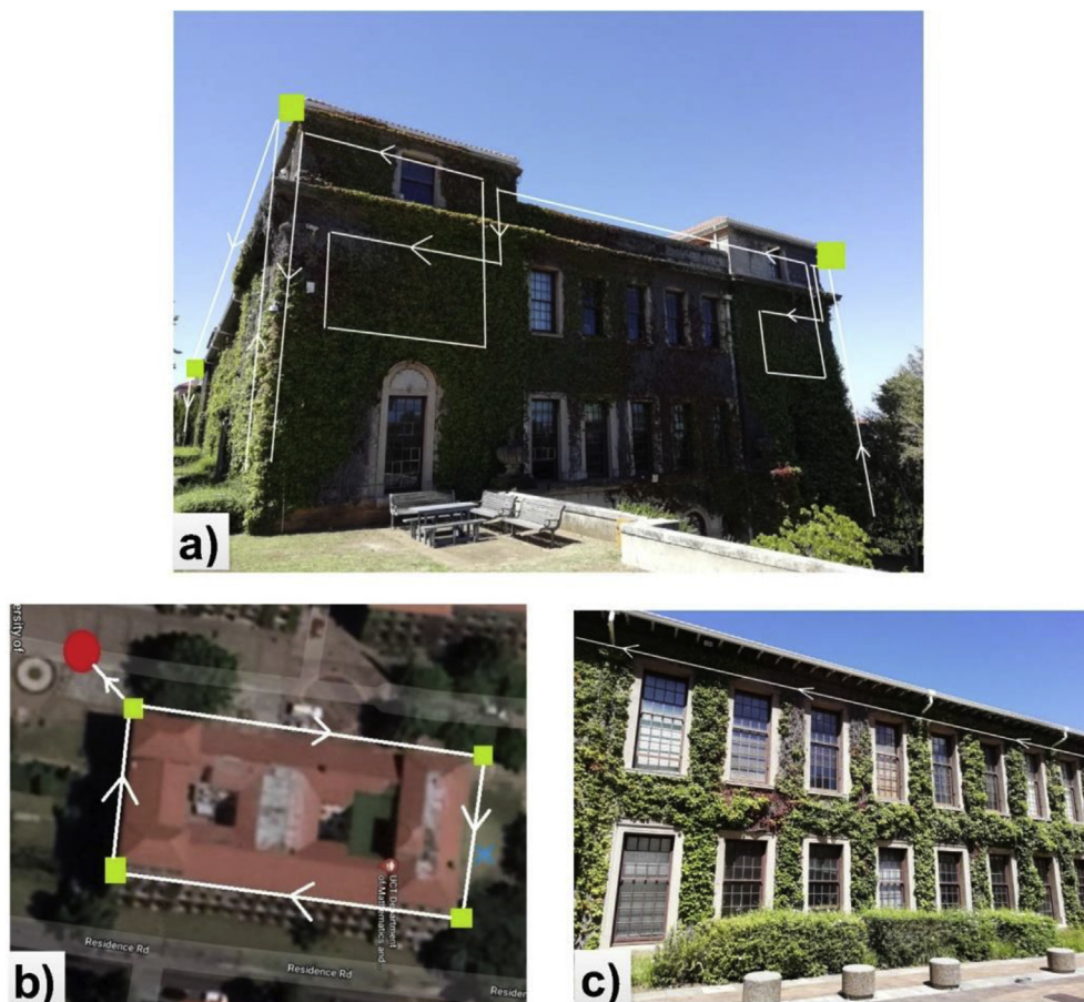
Fig. 2 Images of Building 1, with sample portions of the UAV flight path marked by white lines. (a) Flight paths on a façade. (b) Flight path around the building marked on an aerial view (©Google Maps). The red dot represents one of the staging points on the ground. The blue cross represents a secondary landing site that was kept ready in case of unplanned landing. (c) Flight path along a roof-wall edge.
