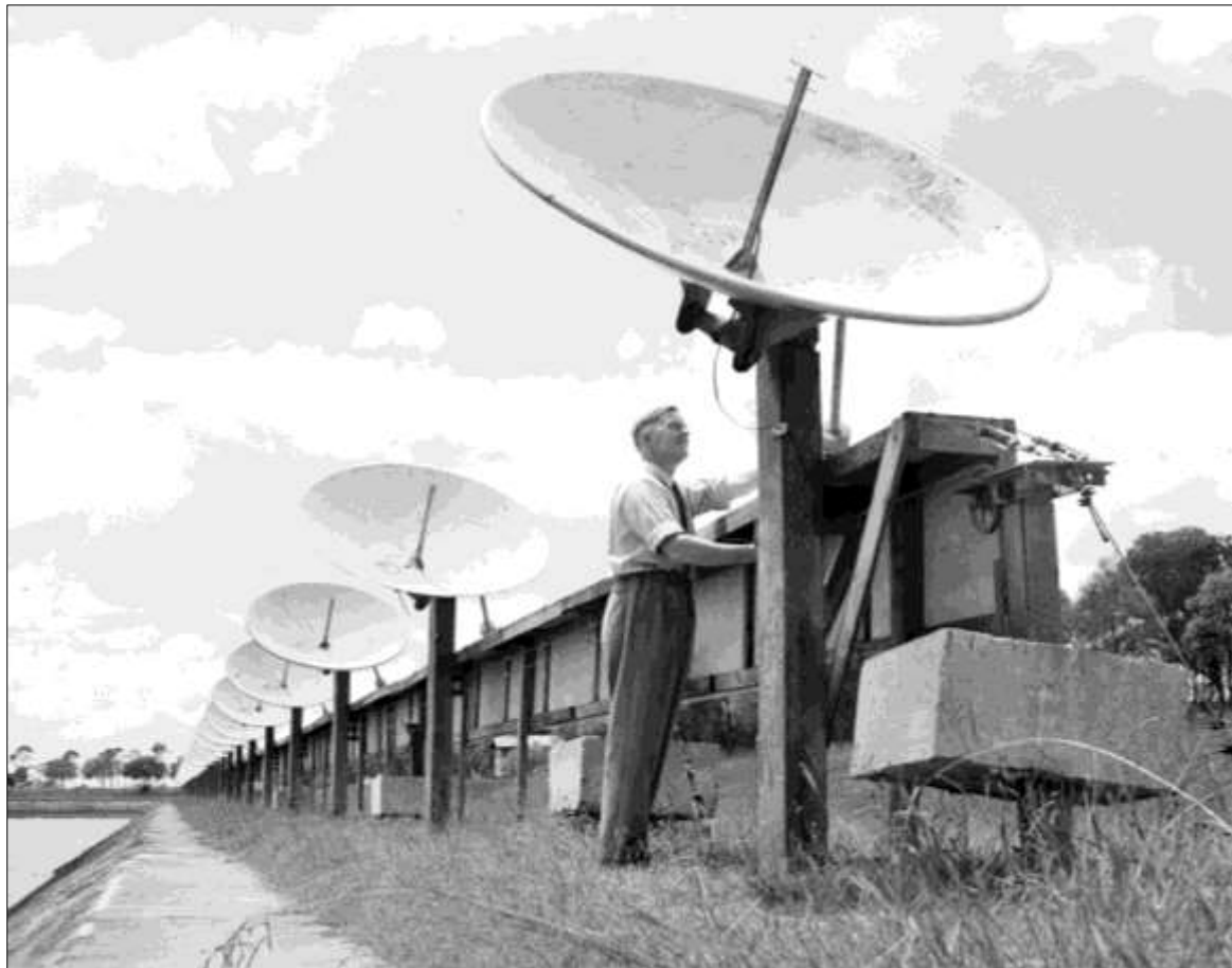
Figure 5: A close-up view, looking east, showing the E–W grating array and Chris Christiansen. The array comprised 32 solid metal parabolic dishes each 1.83 m (72 inches) in diameter and spaced at 7 m intervals (courtesy: RAIA: B2976-1).
