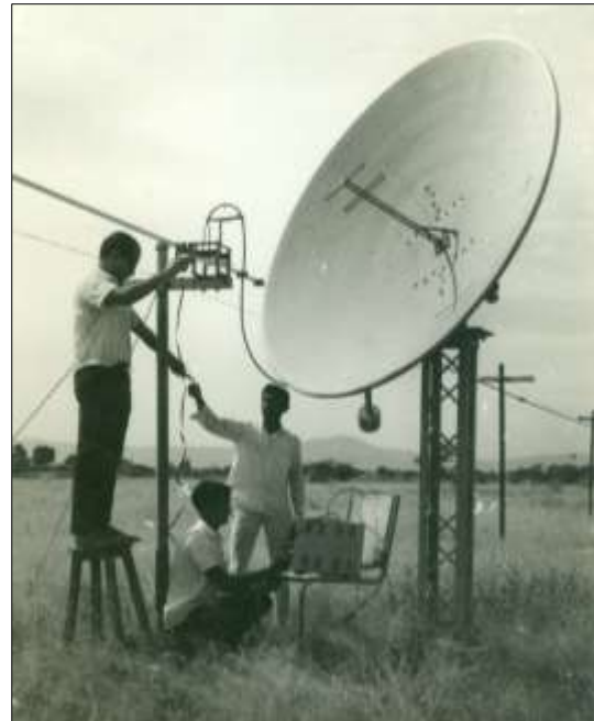
Figure 25 (right): A close-up of one of the Kalyan Array antennas showing J.D. Isloor adjusting the transmission line (courtesy: NCRA Archives).
