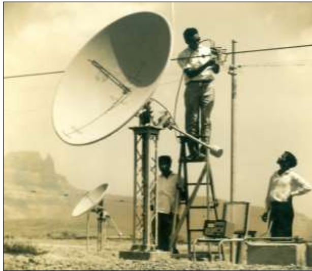
Figure 24 (above): A close-up of one of the Kalyan Array antennas showing the equatorial mounting and support pillar developed by J.D. Isloor. In this photograph V.K. Kapahi can be seen adjusting the transmission line (courtesy: NCRA Archives).
