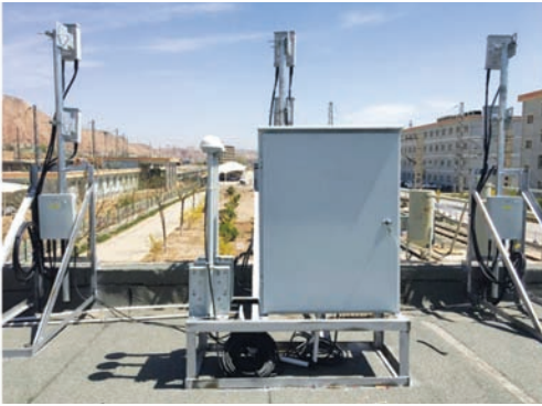
图7 系统部署和应用场景二(无线基站) Fig.7 System deployment and application scenario 2 (wireless base station)
