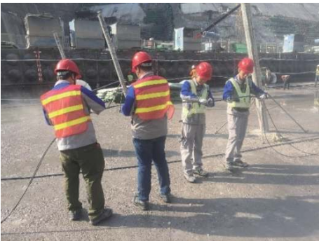
图 2 开仓前待埋光纤双股绑扎施工 Fig. 2 Bifilar binding construction of optical fiber
