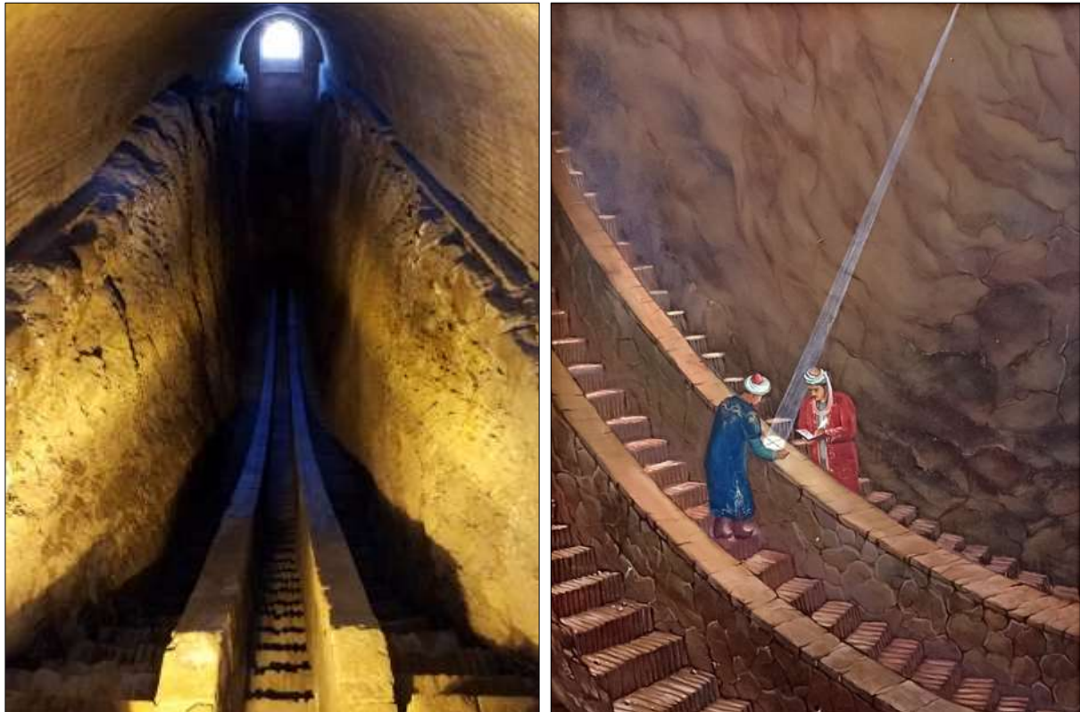
Figure 8: Ruins (left) of the main instrument at the Ulugh Beg Observatory, the 40-meter radius double meridian arc (photograph: Shuhrat Ehgamberdiev), and on the right an artist's depiction of how it was used (courtesy: Museum of the Ulugh Beg Astronomical Institute).
