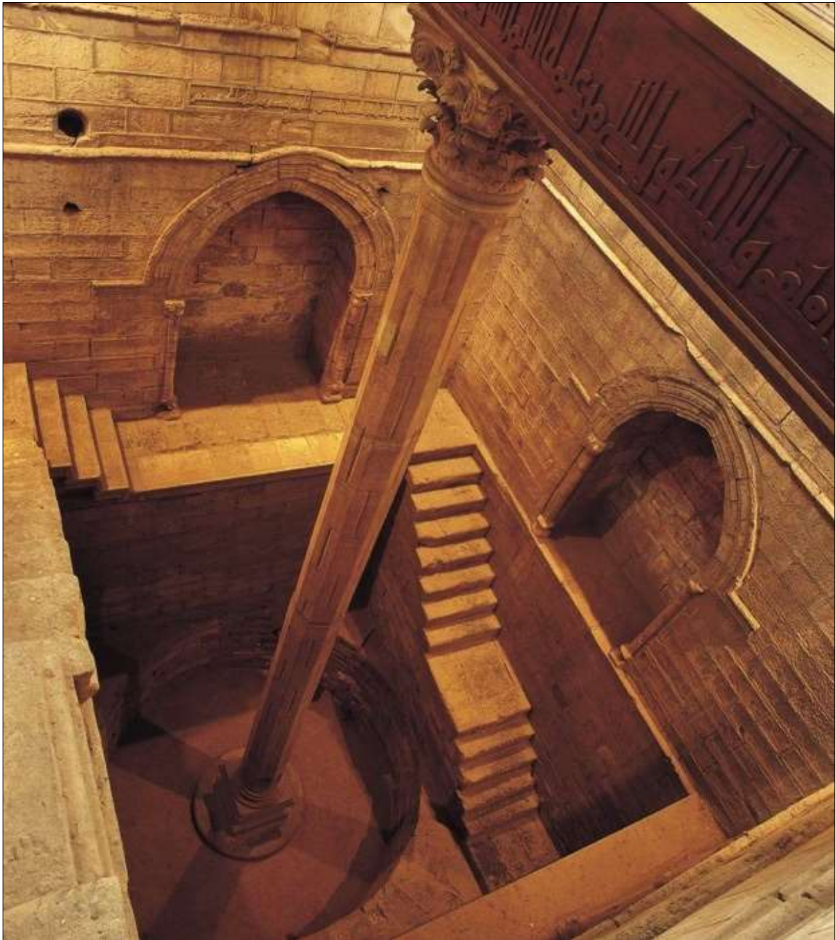
Figure 2: The Nilometer on Rawda Island near Cairo. This was designed to measure the water level during the Nile floods, was used annually to determine the amount of tax levied on the peasants. In 861, the Cairo Nilometer was restored by Ahmad al-Fargani on the orders of Caliph al-Mutawakkil (r. 847–861) (courtesy: A. Akhmedov).
