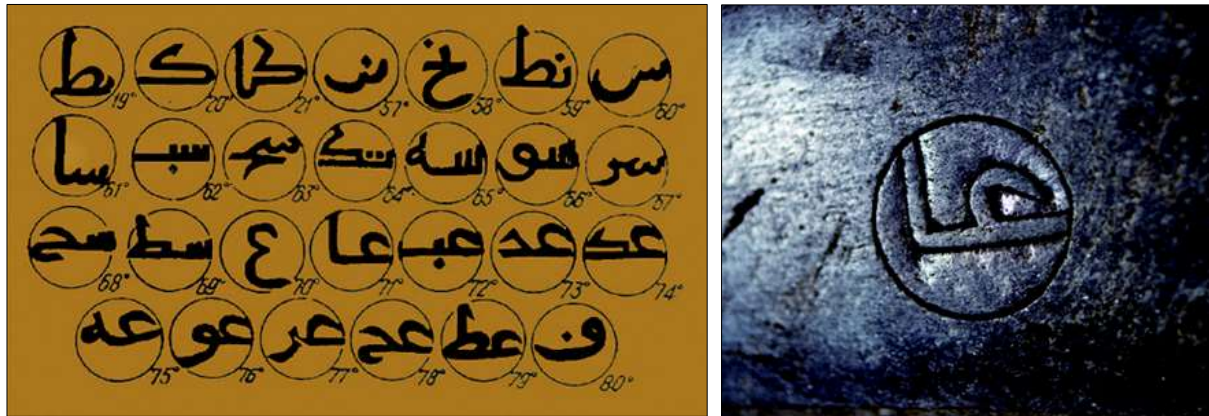
Figure 9: Sketches of degree signs (left) at the surface of the meridian arc and a photograph of the 71° sign (right). The interval of 1 degree on the arc corresponded to 72 cm. With these dimensions, the midday height of the Sun could be determined with great accuracy (source: Sh. Ehgamberdiev).
