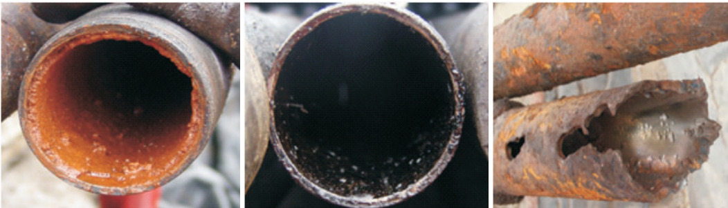
图 2 单元注气三采井油管的结垢腐蚀 Fig.2 Scaling and corrosion of strings in the third round of oil recovery in gas injection wells
