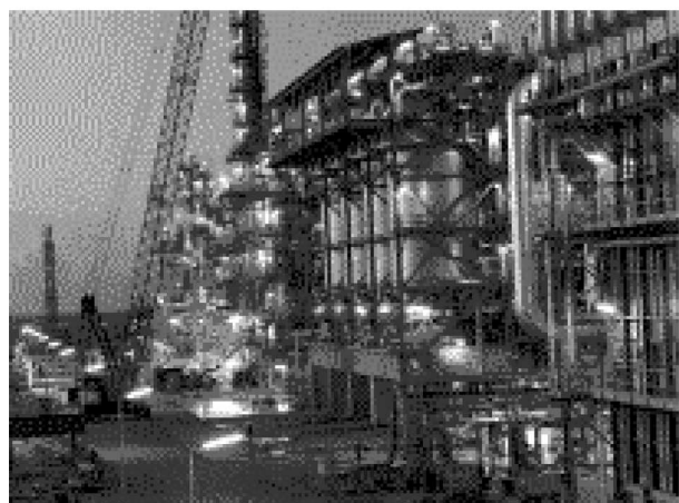
Figure 3. Heavy paraffin synthesis reactors in SMDS plant, Bintulu, Malaysia
