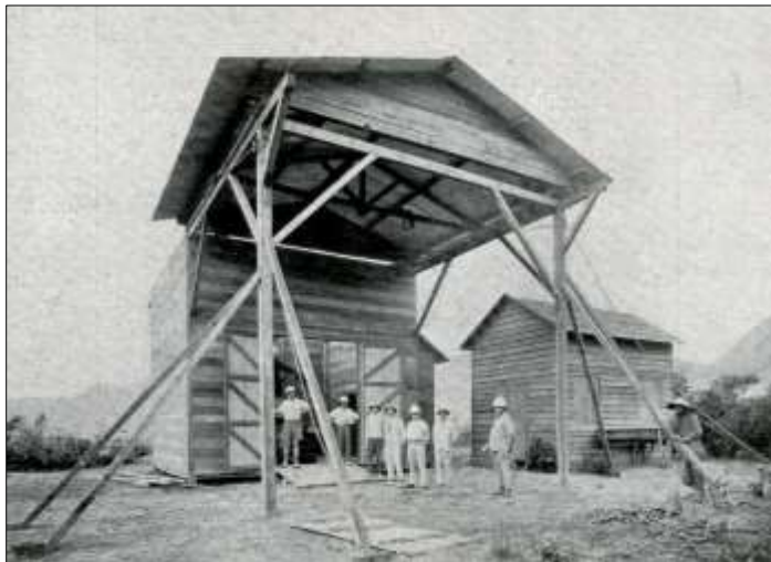
Figure 5 (above): The building for the double equatorial, in front, with its roll-off roof. The smaller building, with a fixed roof, contained the photometry instruments. The people in the photograph could not be identified (after L'illustration of 23 November 1929, Library of Paris Observatory).
