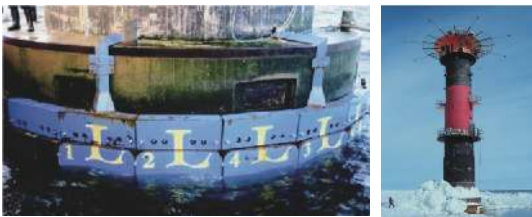
图 5 Norströmsgrund 灯塔及压力板示意图 [43] Fig. 5 Schematic diagram of load panels on Norströmsgrund lighthouse
